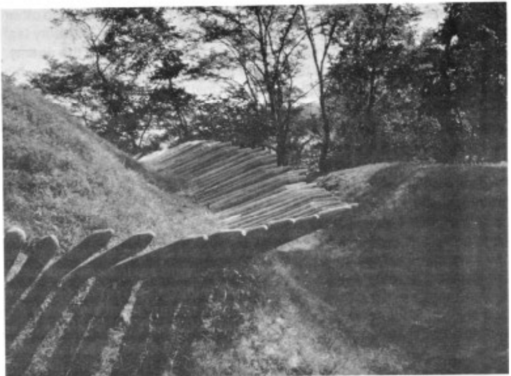
REDOUBT NO. 10. The photographs provide two views of the restoration at Yorktown showing fraisework of the redoubt captured by Americans during the siege.
