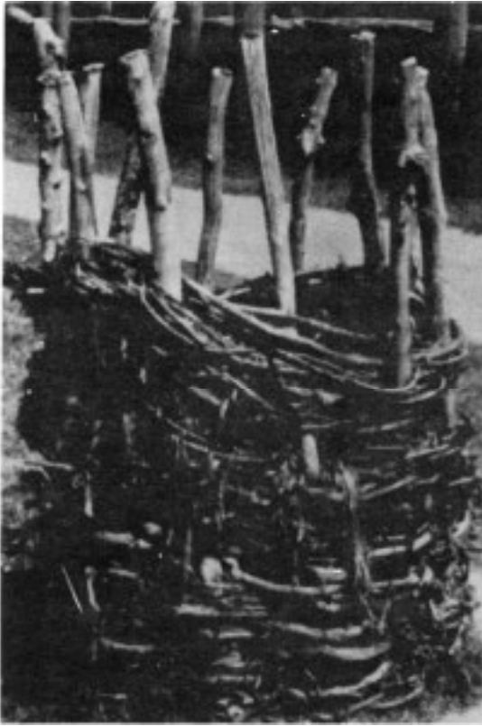
A GABION. This replica of a gabion stands behind the restored American lines at Sara toga National Battlefield Park.
