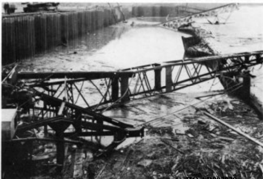
Flooded cofferdam at Emsworth Lock, Ohio River below Pittsburgh, 24 March 1936.
