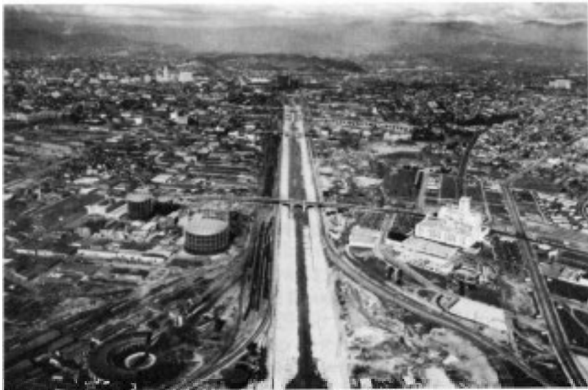
One result of the 1936 Flood Control Act: a concrete flood control channel to help prevent the Los Angeles River from flooding metropolitan Los Angeles. The city hall is in the background at the left. This picture was taken in 1941.
